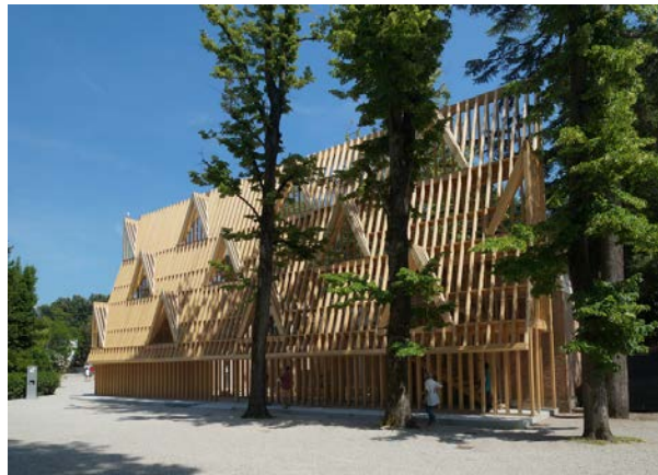
USA: American Framing Foto: Jakob Schoof
