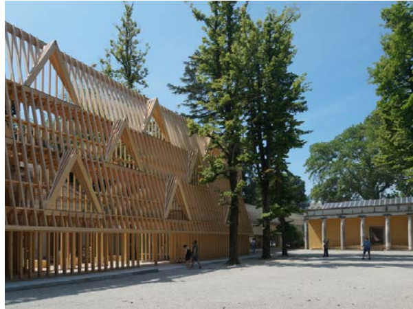
USA: American Framing Foto: Jakob Schoof
