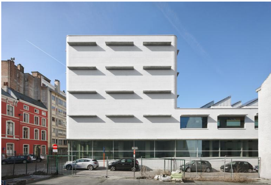
State Archives in Ghent by Robbrecht en Daem Architecten, 2010–2014 (Photo © Filip Dujardin)
