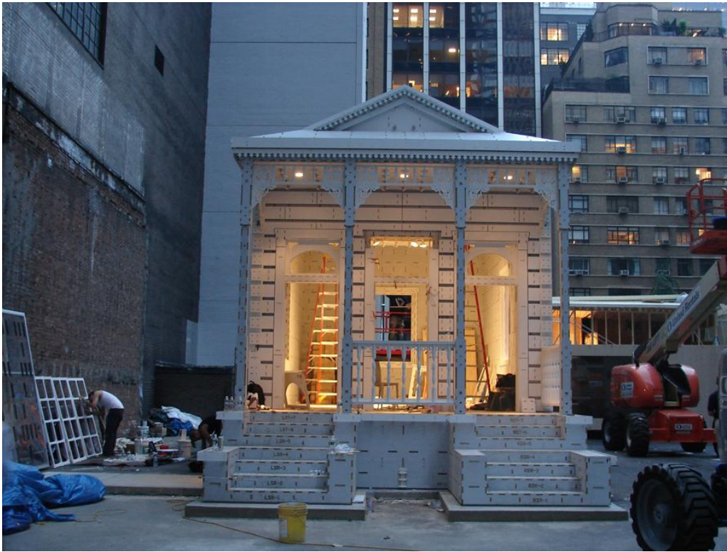
Figure 4. Digitally Fabricated Housing for New Orleans designed by Larry Sass
