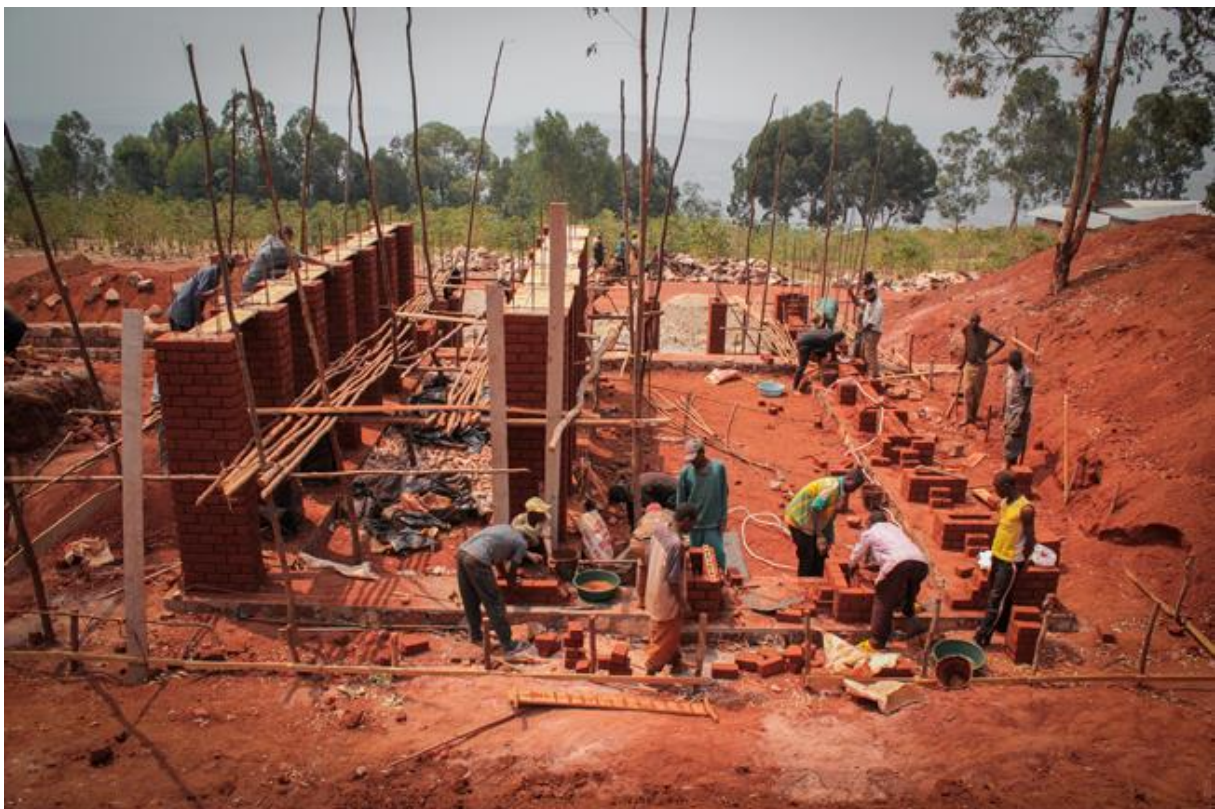
Library in Burundi, built with local materials © BCarchitects&studies
